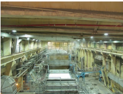
Concrete and Steel Buildings
