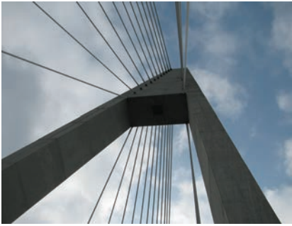
Stay Cable Bridges
