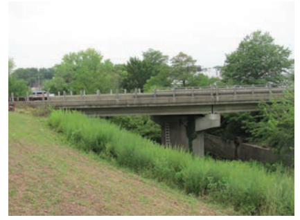
Pre-Stressed I-Beam Bridges
