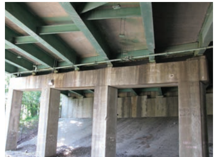
Reinforced Concrete Bridges
