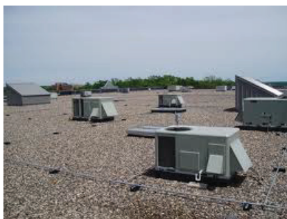
Roofing Leaks (Commercial & Residential)
